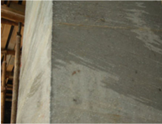
Fig. 5. Concrete pillar wrapped with the YHM-L/204 curing membrane
